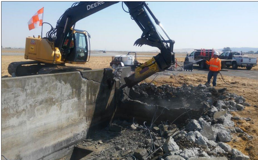
Tearing Down the OWS: A track-mounted hydraulic excavator with a concrete breaker attachment works on one side of an oil-water separator. When complete, the demolition of 11 OWSs will remove unused infrastructure, including two airfield obstructions, and will free up property to support future mission requirements. (Photograph by Lorenzo Lujan [CH2M])
