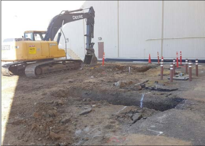
Figure 1: Washboard bioreactor excavation. Photo Credit: Jacobs
