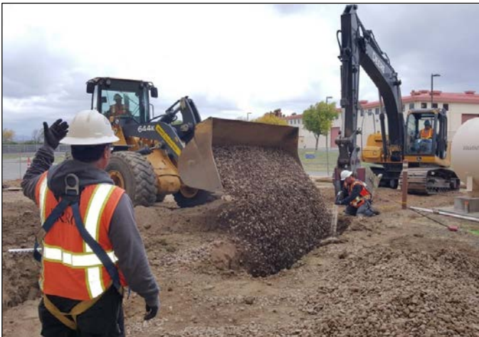
Figure 2: Backfilling the excavation with a mixture of gravel and amendments. Photo Credit: Jacobs
