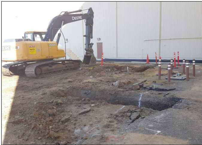
Figure 1: Washboard bioreactor excavation. Photo Credit: Jacobs
