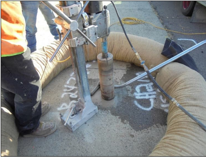
Photo 3: Concrete coring in 2016, in preparation for drilling a soil boring. Photo Credit: Jacobs
