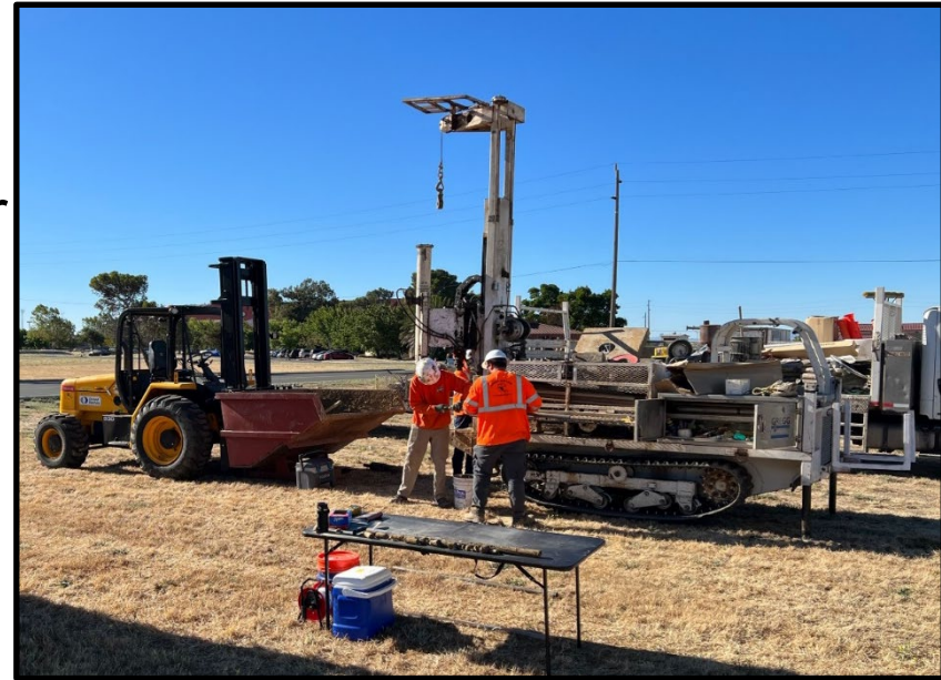
Oneida Team installing a groundwater monitoring well
