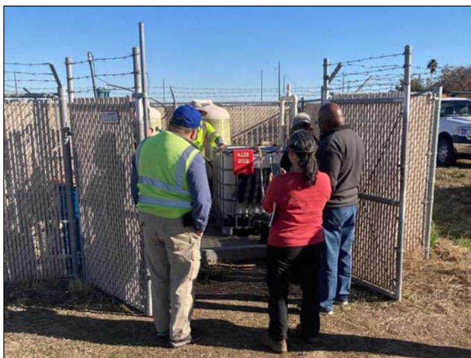
RAB members at the smallest of the three treatment plants visited. This plant is 100 percent solar-powered and treats about 125,000 gallons of trichloroethene-impacted groundwater monthly.
