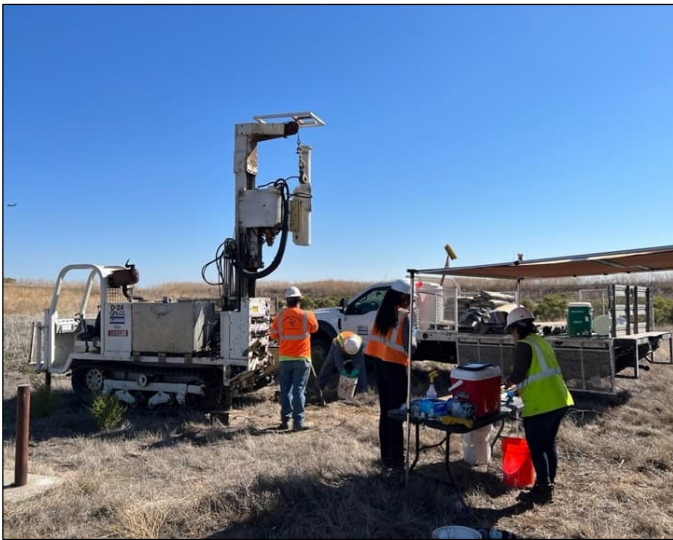
Oneida project geologists direct monitoring well installation and collect soil samples during Field Event #2.
