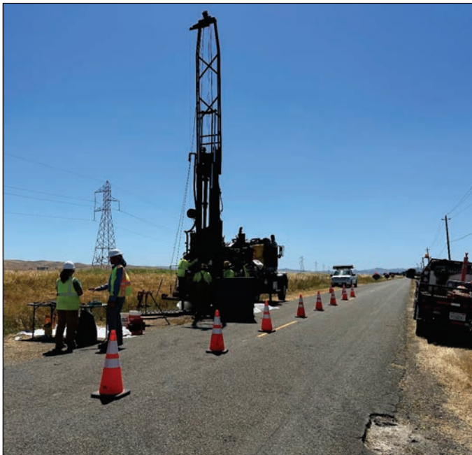
Figure 2: Field team reviewing soil cores as drillers begin constructing a monitoring well using hollow-stem augers. Photo Credit: Oneida.
