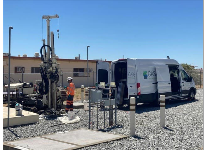
Figure 3. DPT drilling with UVOST/MIP support vehicle. Photo Credit: Jacobs
