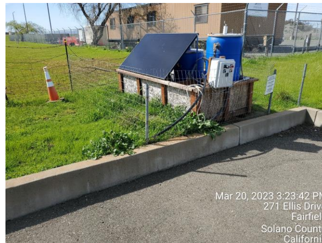
•Solar Power Organic Carbon Treatment System at DP039
