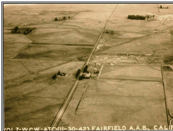
Figure 8. Early construction at Fairfield-Suisun Army Air Base in November 1942 looking east. The road in the center is today's Travis Avenue.
