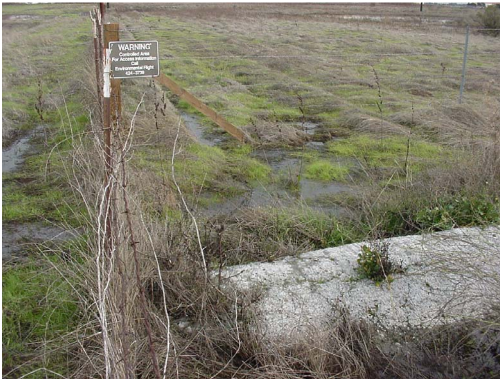
Photograph 6: Start of LF044 Fencing and Berm.
