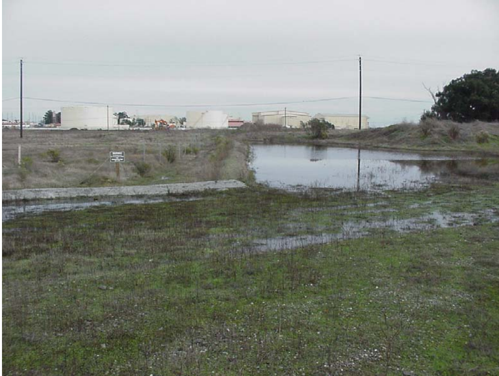
Photograph 7: LF044 Berm, Facing East.
