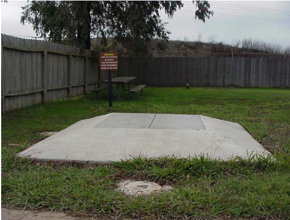
Photograph 1: Controlled Area at DP039.
