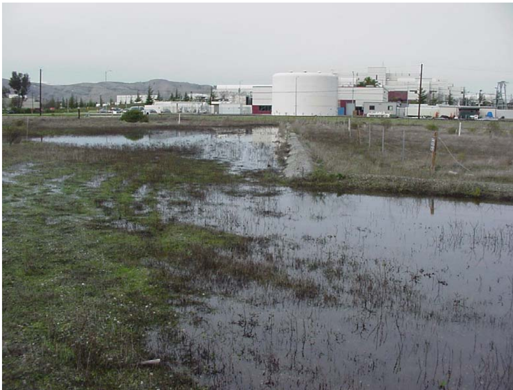
Photograph 8: LF044 Berm, Facing North.
