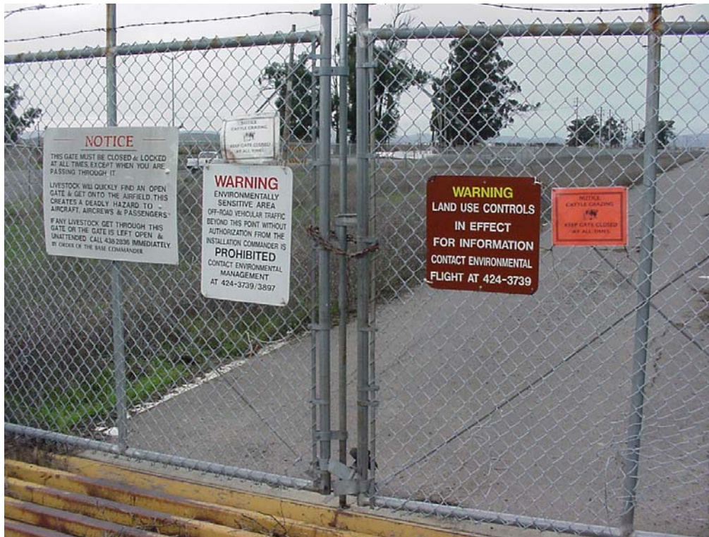
Photograph 9: Fence Access to SD045. Warning sign is posted on gate entry.
