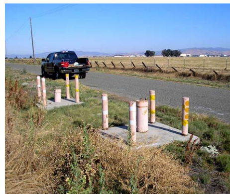
Now you see 'em, now you don't: Two sets of off-base monitoring wells along Creed Road were decommissioned at the request of the county engineering office. The four wells were no longer used by the base, and their removal improved road safety along the roadway shoulder.
