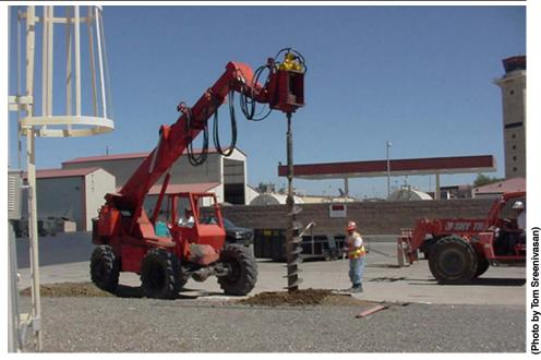
Wall Drilling: Site workers use an auger rig to install footings for a sound wall at the Central Groundwater Treatment Plant. The finished wall reduces the ambient noise from the water treatment equipment and meets base architectural standards.
