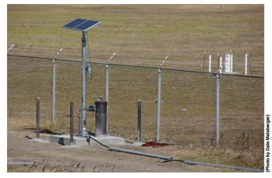
**Remote Pumping Station:** Two extraction wells use solar arrays as a source of electrical power to bring contaminated water up from the subsurface and to transport it to a local treatment plant. An off-base monitoring well sits north of the base boundary.
