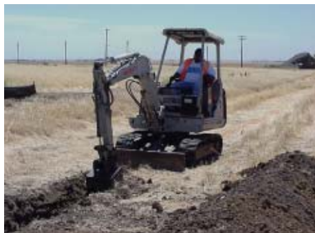
Extraction well installation near CAMU.
