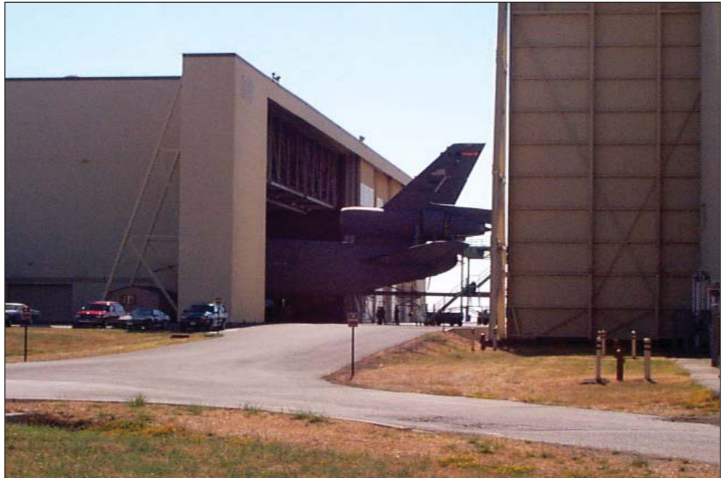
Hangar at Work: Aircraft maintenance and repair takes place in a number of hangars on Travis AFB. Known as Facility 811 (site designation SD034), this is one of 12 Travis AFB soil sites that does not need an active cleanup remedy to protect human health and the environment.
