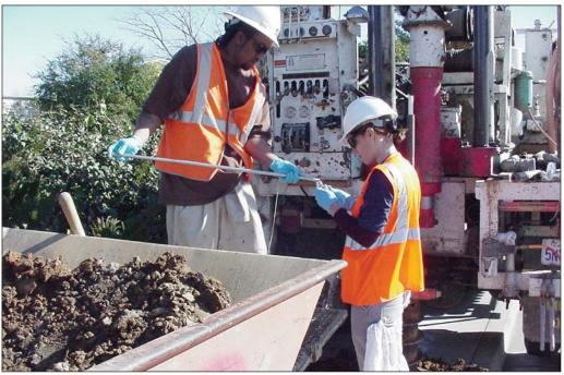
**Easy Does It:** Field team members from CH2M HILL, an environmental consulting firm, carefully collect groundwater samples from a soil boring, using a bailer. The water samples will be analyzed for petroleum constituents. Laboratory analysis results will be used to identify the contaminants.
