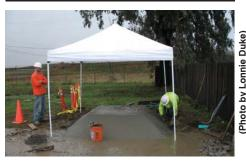
Construction engineers battle wind and rain to put finishing touches on a protective vault for a new Dual-Phase Extraction well at a groundwater site.
