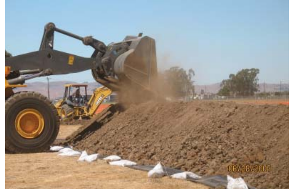
The heavy equipment operator carefully places contaminated soil on top of a soil pile to minimize the creation of airborne dust.
