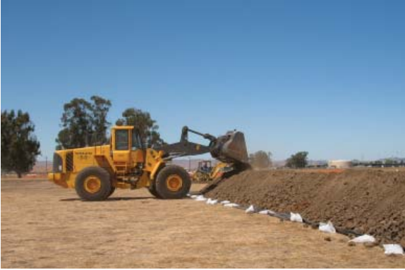
Contaminated soil is placed on top of plastic sheeting in long rows and will be covered to prevent wind erosion.
