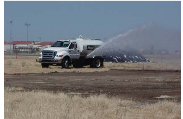
A 2000-gallon capacity water truck sends a stream of water across a work zone to minimize the transport of contaminated airborne dust away from a cleanup site.
