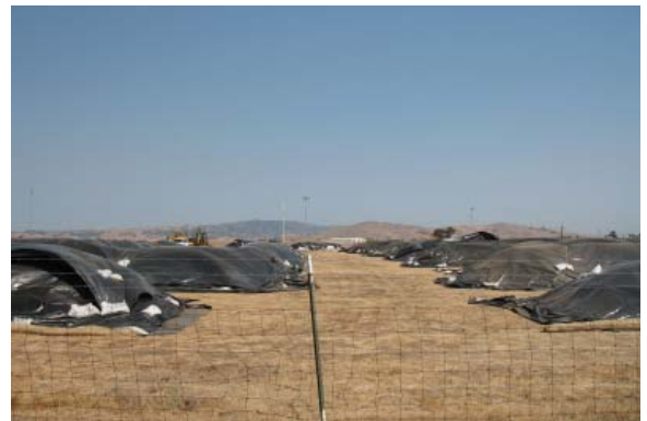
Sand bags are placed on top of plastic sheeting that is covering piles of contaminated soil.
