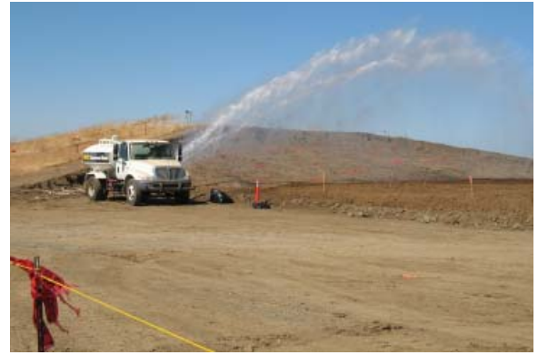
A water truck sends a stream of water across contaminated soil at an on-base soil repository to assist with its compaction.
