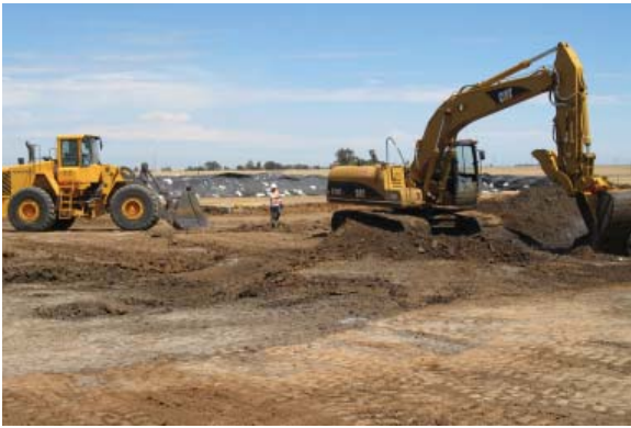
A field technician with an XRF tool directs two heavy equipment operators to excavate soil in discrete locations. XRF lets the field team accurately identify the extent of contaminated soil.
