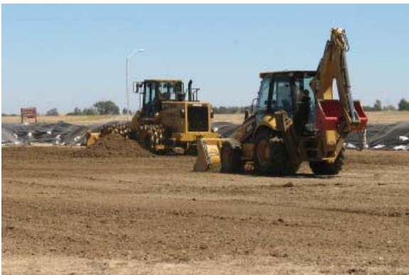
A backhoe and compactor move backfilled soil across an excavation void, restoring the site to its original topography.
