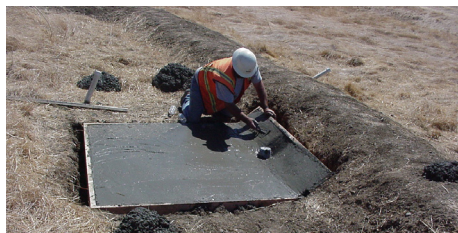
A field technician from Shaw Environmental finishes his work on a surface water drain to the Corrective Action Management Unit.
