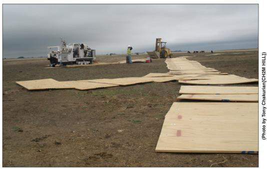
**Walking the Plank:** Field technicians created a roadway of wood panels across a sensitive environmental habitat to allow vehicles to reach groundwater sampling locations. Precautions such as these allow groundwater samples to be collected without damaging the overlying soil and vegetation.
