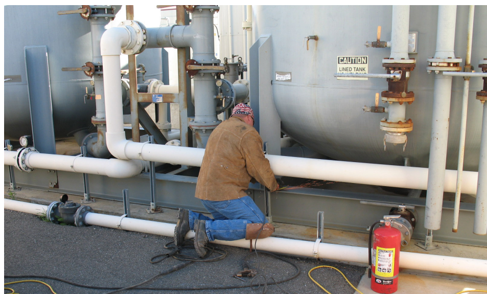
Patching the Tank: A field technician conducts a repair on one of two 20,000 pound granular activated carbon canisters at the Central Groundwater Treatment Plant on Travis AFB. Because of their many years of service, the costs to maintain the four groundwater treatment plants on base are expected to increase over time. (Photo by Glenn Anderson)
