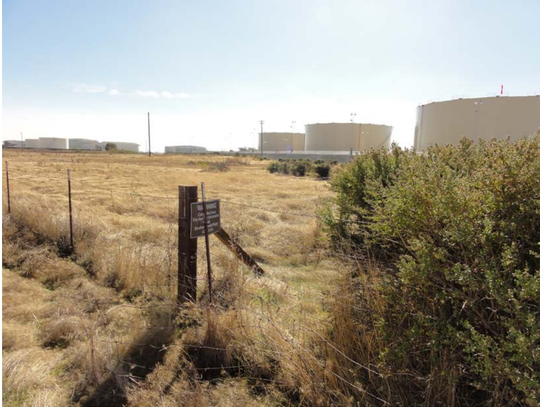
Photograph 11: North Side of LF044 Fence
