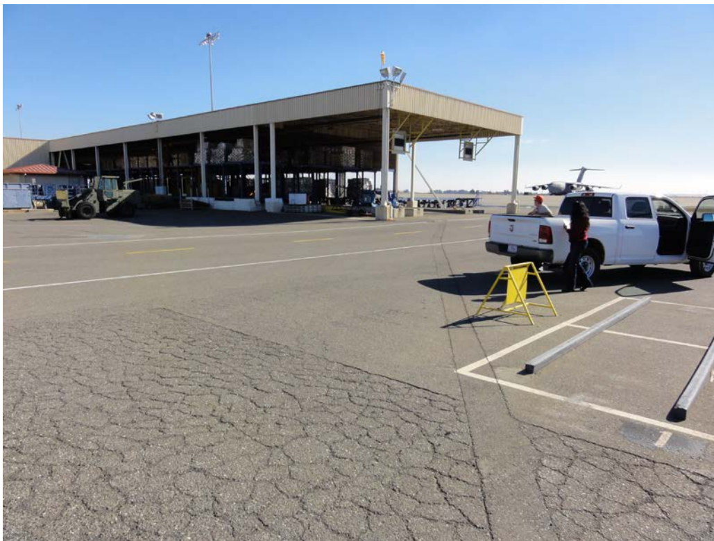
Photograph 6: Controlled Area on Southwest Side of SD037
