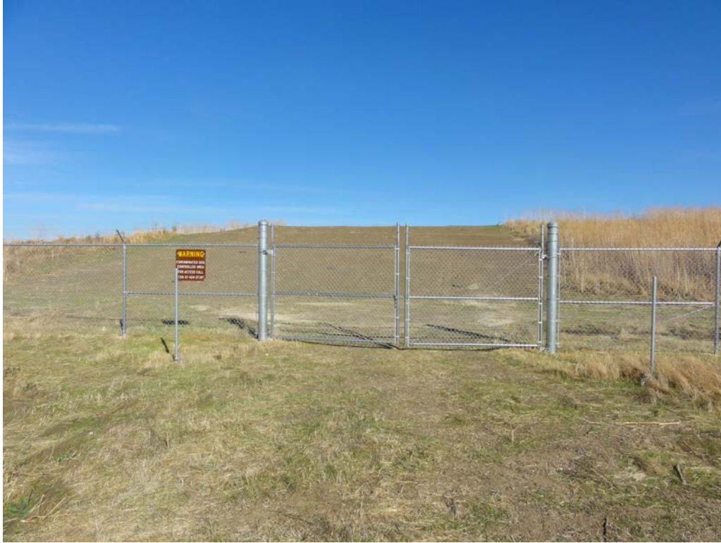
Photograph 15: Northwest CAMU Gate after Lysimeter Removal
