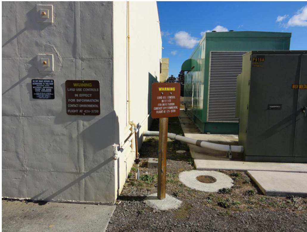
Photograph 9: Generator Pad and Warning Signs at SD043. Stanchion of Former Pad with Leaking Transformers is visible just behind the warning sign post.
