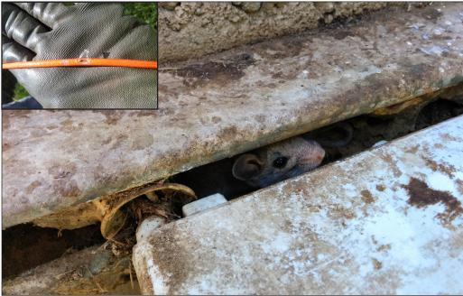
**Varmint in the Vault:** A field mouse is spotted in an extraction well vault that supports the cleanup of contaminated groundwater. Often, small mammals will chew on the electrical wire that connect pumps to treatment systems, resulting in shutdowns and costly damage (shown in the inset).
