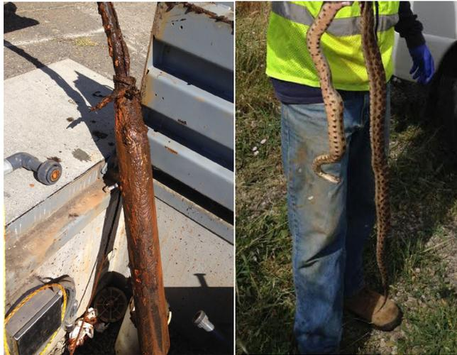
**Fieldwork Follies:** Suspended sediment in groundwater can coat an extraction pump (shown on the left), causing excess wear and tear and often leading to early pump failure. When field technicians discover the mechanical problems and visit the site to conduct repairs, they are often greeted by the local inhabitants, such as the non-poisonous snake shown in the right photo. [Photos by Eric Phelps (CH2M HILL)]
