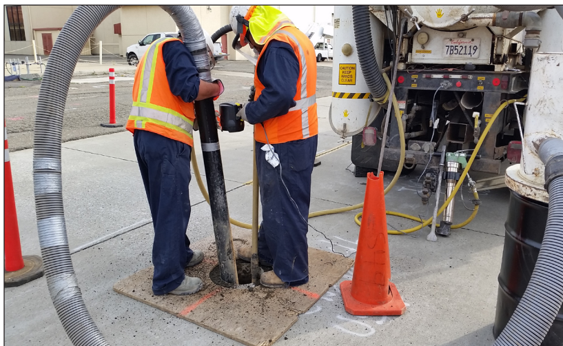
Don't Cut My Cable: To prepare for the installation of a monitoring well, field technicians remove the upper soil layers, using air knitting equipment. This technology uses compressed air and vacuum excavation to safely uncover any buried utilities without damaging them. [Photo by Erin Crandall (CH2M HILL)]
