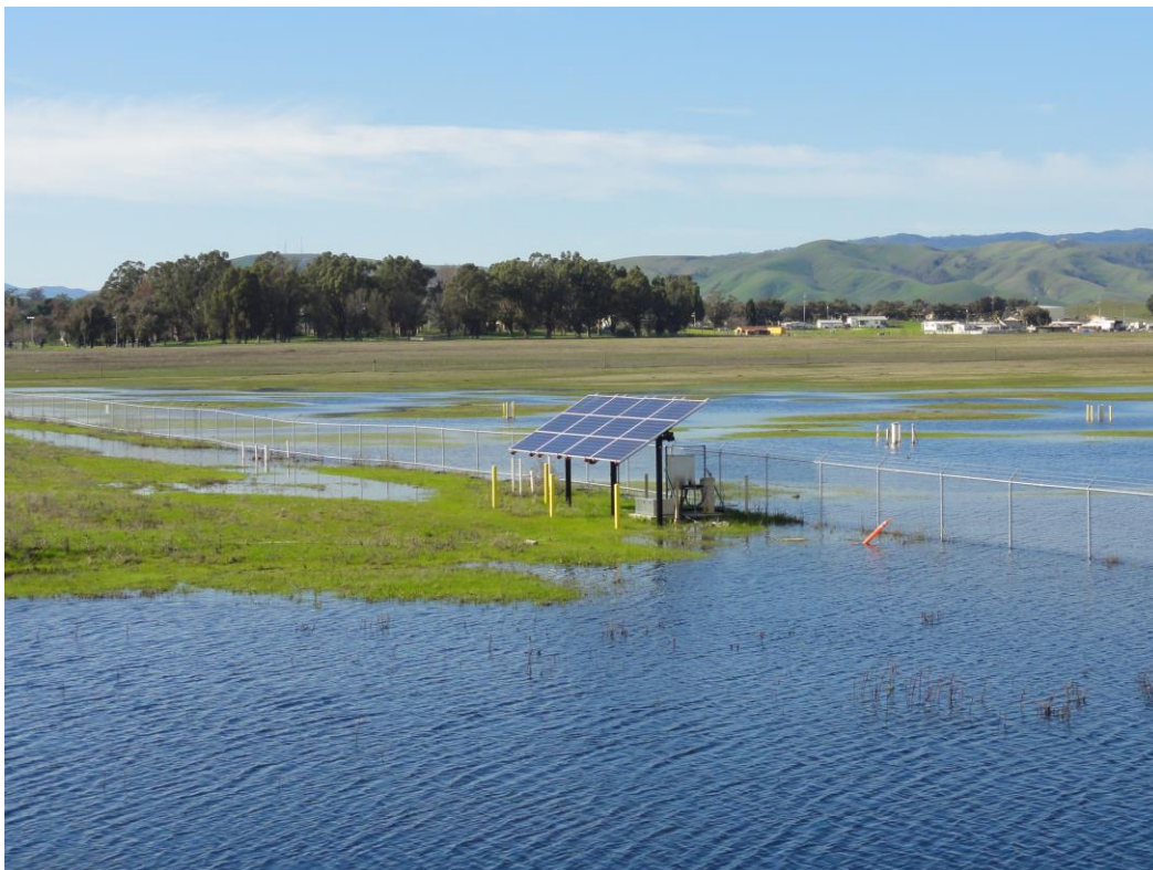
Photograph 10: Close-up of Solar Powered Extraction Well at LF007C [NW]
