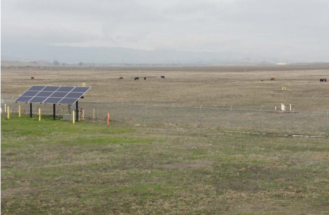
Photograph 9: View of LF007C Extraction/Monitoring Well Network [NW]
