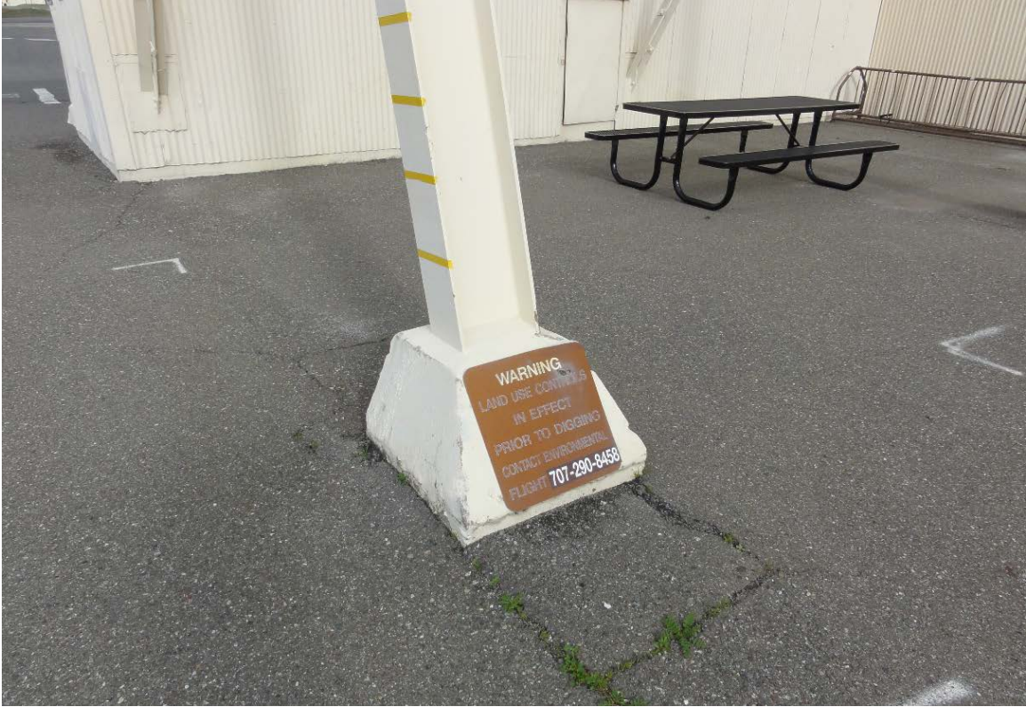
Photograph 21: Warning Sign at Controlled Area on West Side of SD033 [NE]
