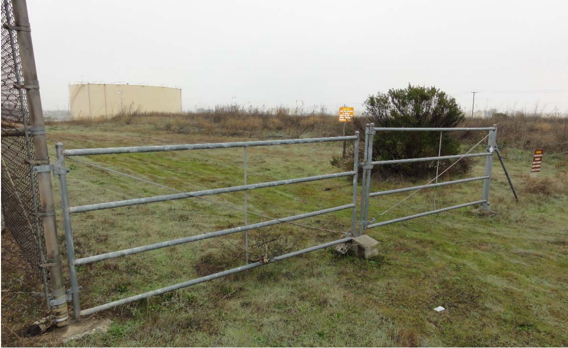
Photograph 35: Gate and Warning Sign on South Side of LF044 [NNE]
