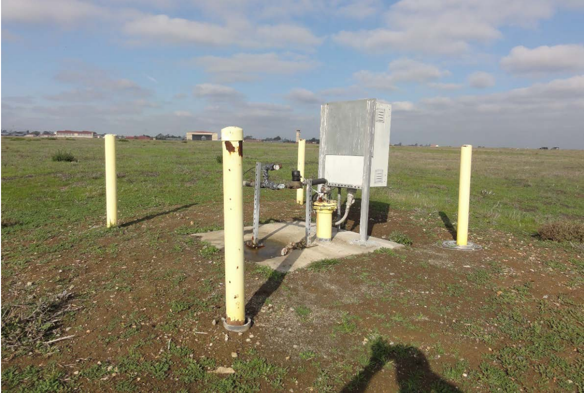
Photograph 17: View of SS029 Extraction Well [N]
