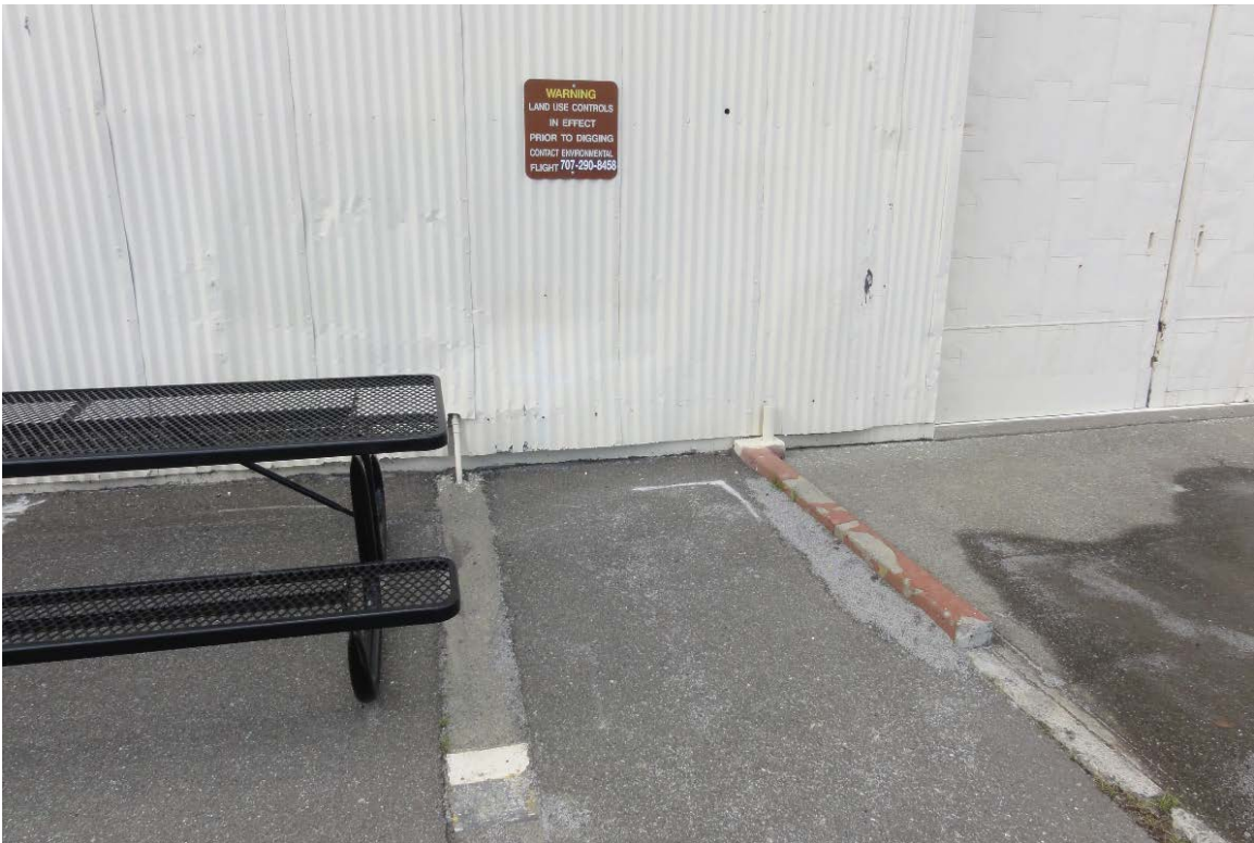
Photograph 20: Warning Sign at Controlled Area on East Side of SD033 [W]
