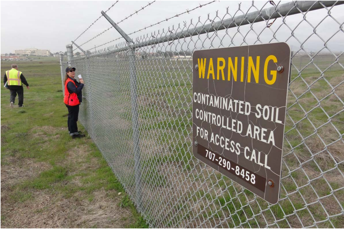
Photograph 7: Southeast CAMU Gate with Warning Sign [NW]
