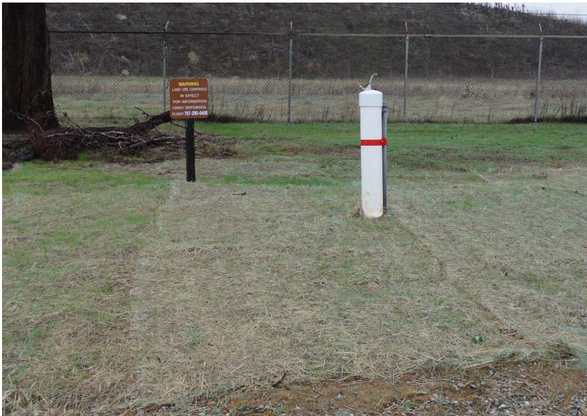
Photograph 28: Controlled Area at DP039 (Bioreactor) [W]
