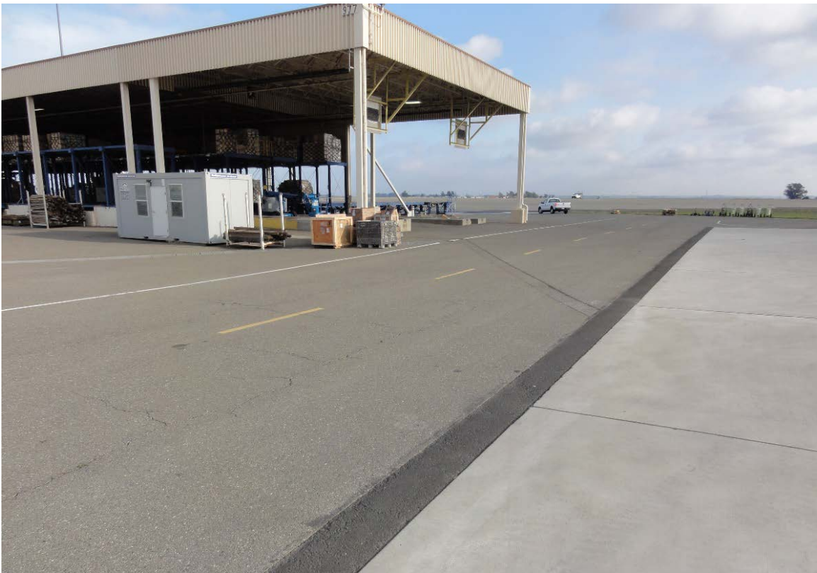
Photograph 26: Controlled Area on Southwest Side of SD037 [SE]
