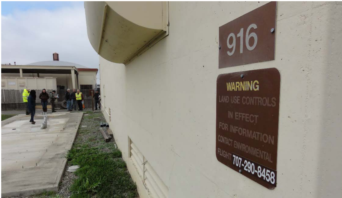
Photograph 31: Warning Sign near East Side of SD043 [W]
