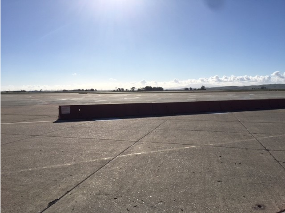
Photograph 39: Former SD032 Location [S]
