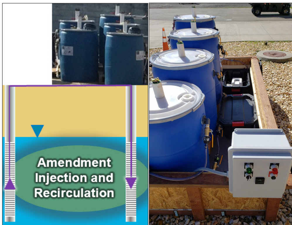
From Design to Production: The schematic diagram on the left shows the components of the SPOC system. Extracted groundwater picks up dissolved organic carbon when it moves through the blue drums and is slowly reinjected back into the ground. The photograph on the right shows the relatively simple equipment layout of the SPOC system. (Diagram by Jeff Gamlin [Jacobs Engineering]) (Photograph by Angel Santiago [AGEISS])
