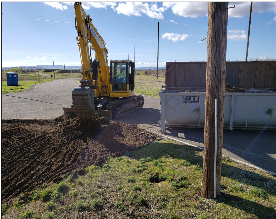
Taking off the Top Layer: A heavy equipment operator places surface soil into a bin as part of the cleanup of polycyclic aromatic hydrocarbon-contaminated soil at the former Railhead Munitions Staging Area. The contaminated soil will be sent by truck to an off-base landfill for disposal. After clean soil is used to restore the site to its original condition, it will be ready for closure. (Photograph by Angel Santiago)
