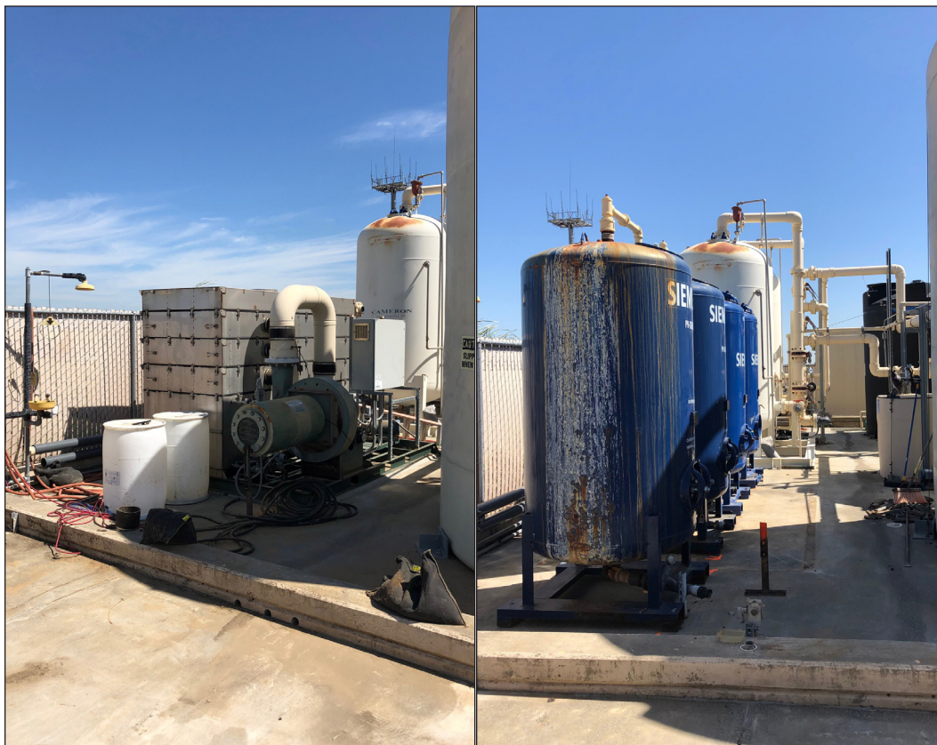
Before and After: Significant changes have been made to the South Base Boundary Groundwater Treatment Plant to make it more efficient and increase its lifespan. The left photograph shows the old air stripper that was shut down because of rising operational costs. The right photograph shows two new and two used activated carbon canisters that will improve plant performance. (Photographs by Gene Clare)
