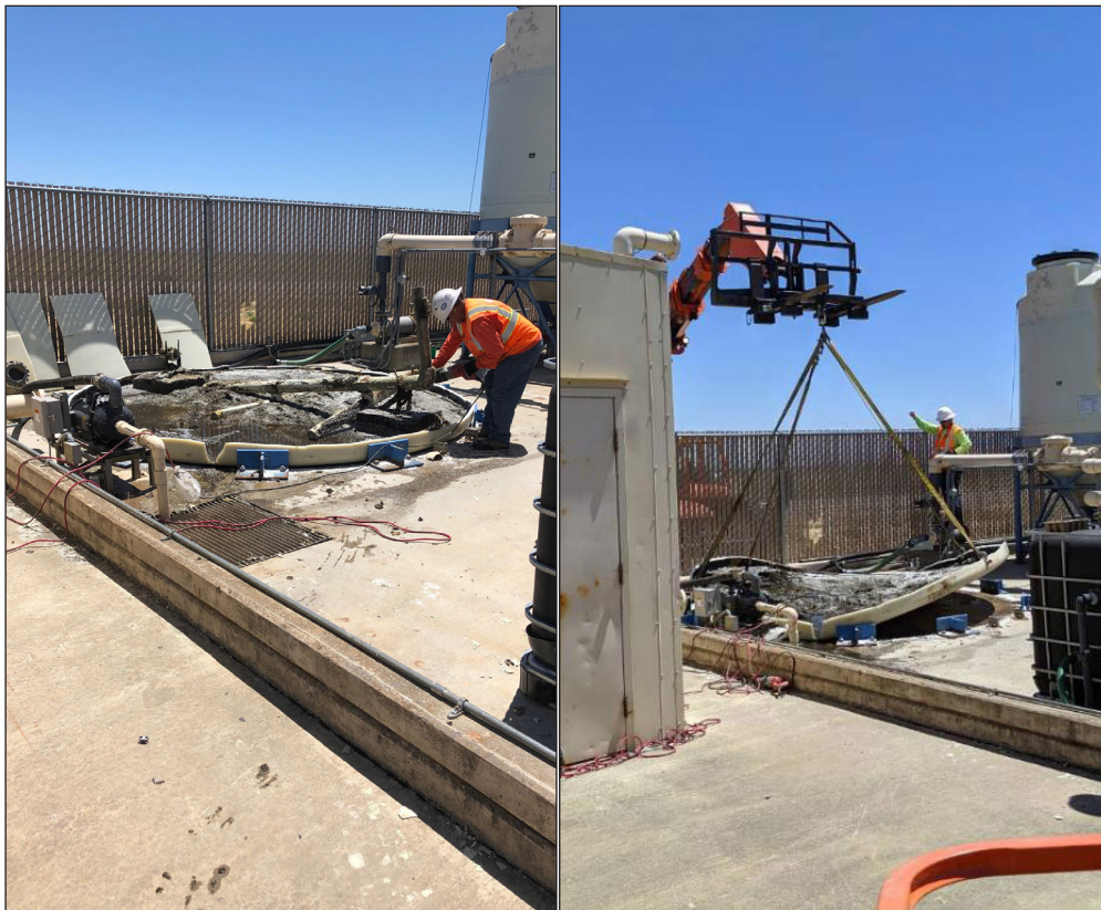
Bottom's Up: Field engineers finish the deconstruction of the treated water tank at the South Base Boundary Groundwater Treatment Plant by lifting the tank bottom from the concrete floor. The left photograph shows the tank after the sides have been removed. The right photograph shows the heavy equipment used to lift the tank bottom off of the treatment plant floor. For more information about this project, please read the July 2019 Guardian edition. (Photographs by Gene Clare)
