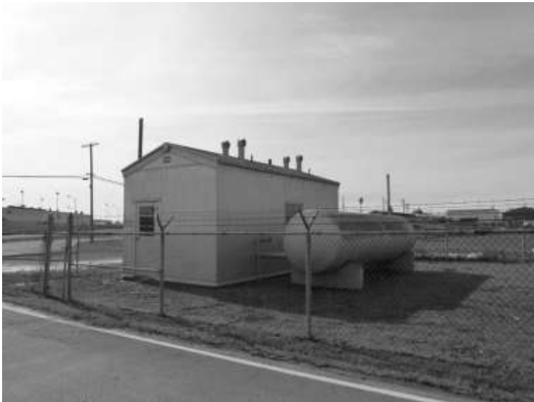
Northeast oblique (ERDC-CERL, January 2012)
