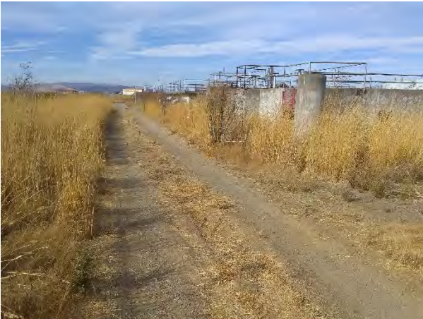
View showing infrastructure to be demolished
