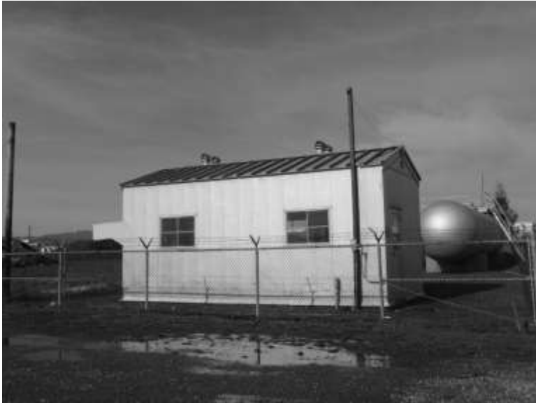
South elevation (ERDC-CERL, October 2011)
