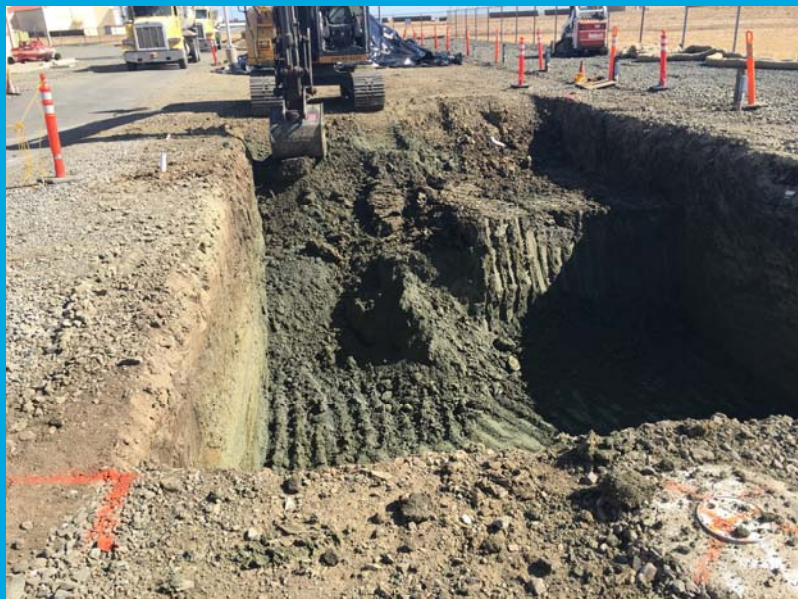
Excavation of Fuel Contaminated Soil
