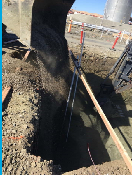
Drywall and Gravel Backfill
