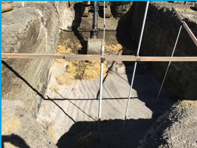
Backfill with Gravel, Drywall, Straw, and Pyrite
