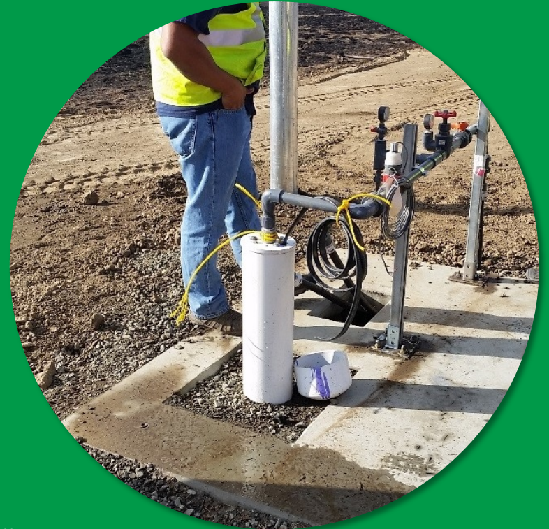
Photo of new FT005 extraction well installation in 2015
