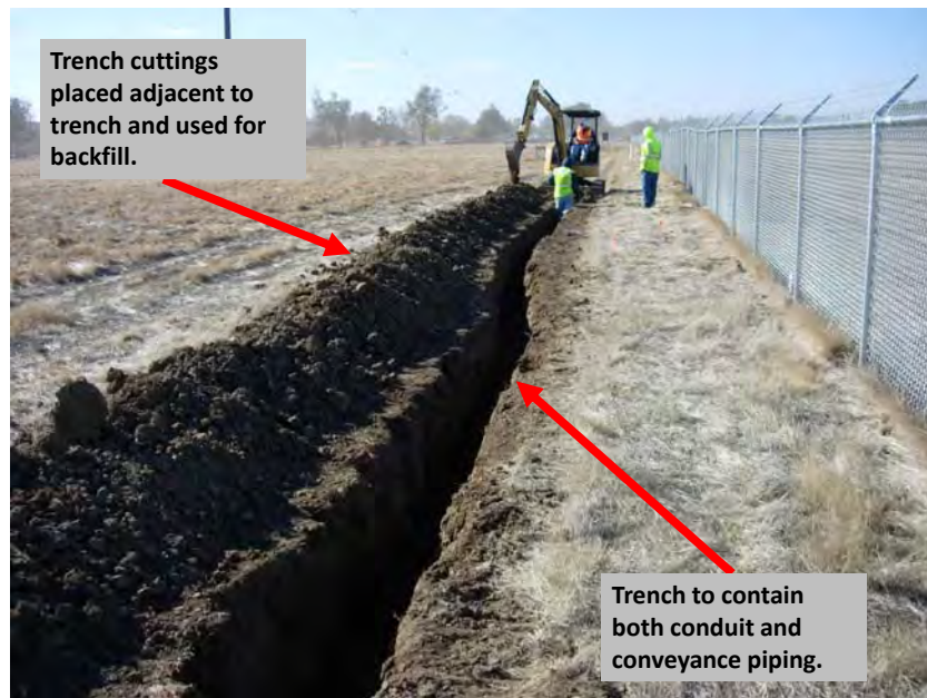
Trenching along the base fence line
