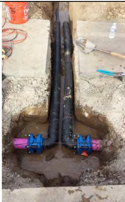
Small diversion for the new treatment system discharge location
