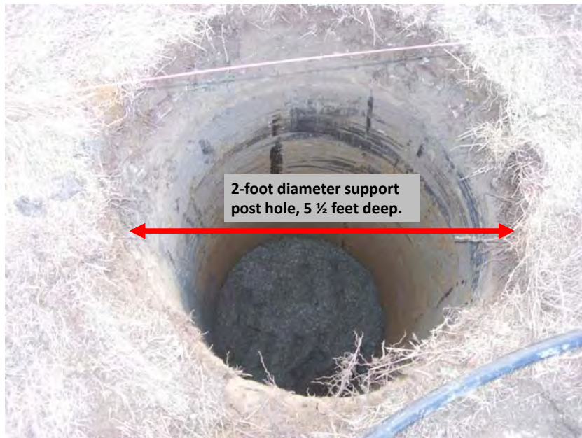
Post hole for solar array support post – three in total
