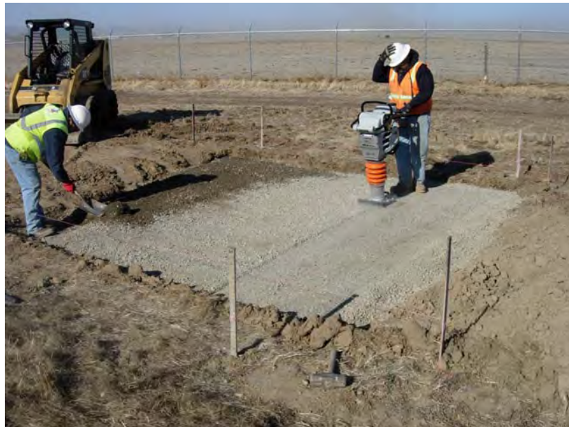
Preparing the treatment system containment pad
