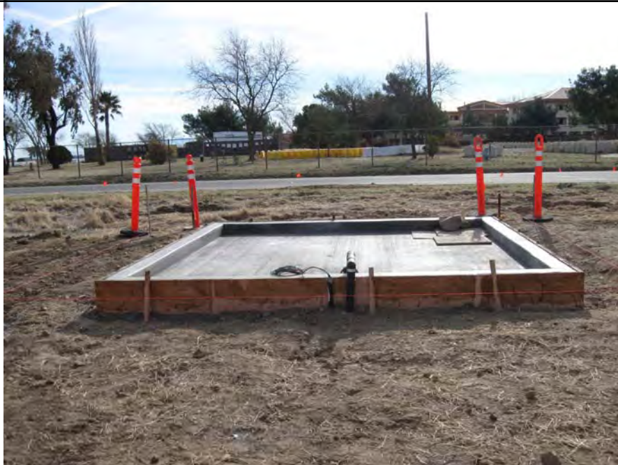
Completed treatment system containment pad
