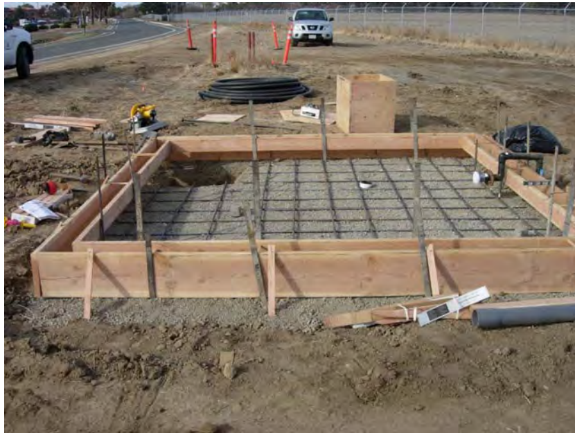
Almost completed the treatment system containment pad form
