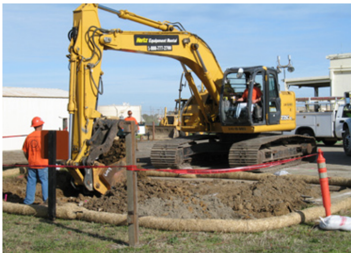
Heavy equipment operators excavate the area around a former battery acid neutralization sump to prepare for the installation of an in situ bioreactor.
