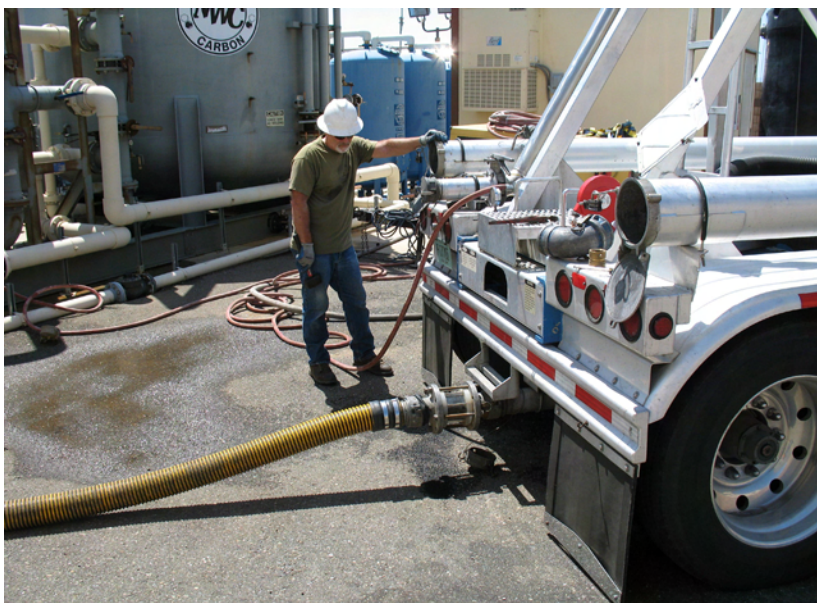
Pumping Carbon: A specialist in granular activated carbon monitors the flow of fresh carbon into one of two 20,000-pound groundwater treatment canisters. The canisters will take the place of an ultraviolet oxidation system that is no longer cost effective at removing organic compounds from groundwater.
