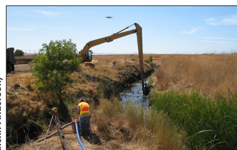
In the background, a long-arm excavator removes contaminated sediment from Union Creek. In the foreground, a field technician checks on the performance of a gas-powered pump that is dewatering the contaminated portion of the creek.
