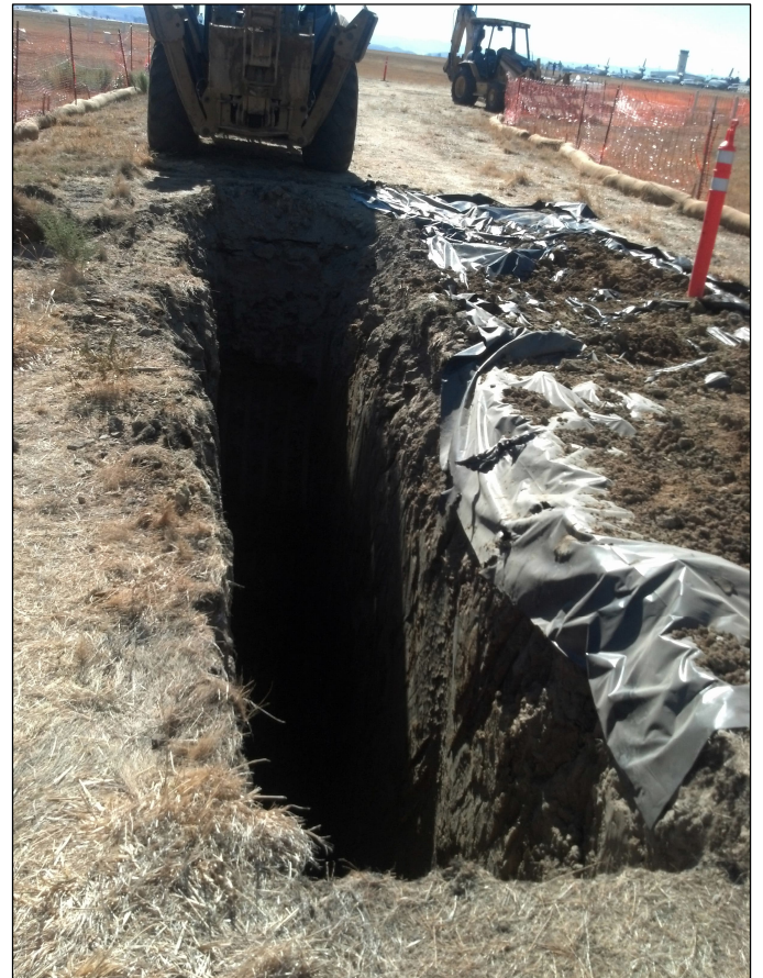
Figure 4. Photo of a fully excavated bioreactor trench. (Photo credit: Jacobs)
