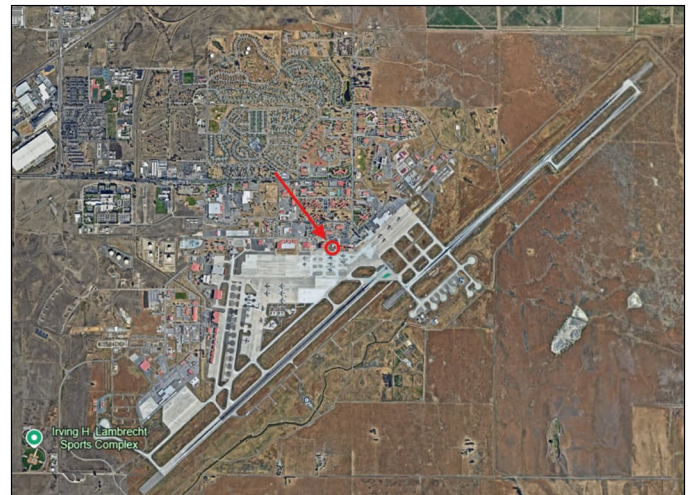
Location of the Central Groundwater Treatment Plant within Travis AFB (click on image to enlarge). (Image credit: Jacobs)
