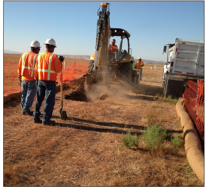
Figure 3. Photo of the excavation of a bioreactor trench. (Photo credit: Jacobs)
